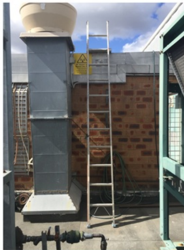
Figure 36. Roof top access via ladder
