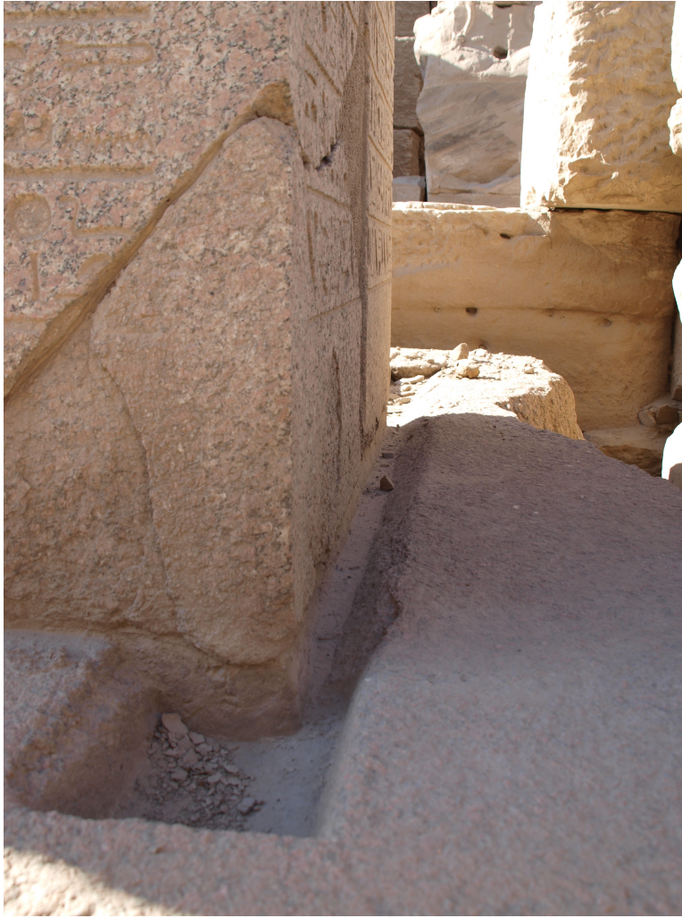
Fig 2.11 The base of the southern obelisk in the courtyard between Pylons Four and Five. The groove used to erect the obelisk is visible of the northern edge. Photo: G. Smith.
