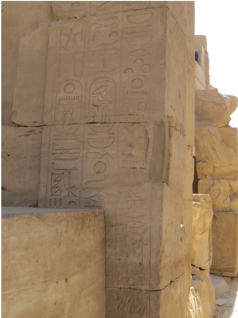
Fig. 4.11 The northern doorway of the chamber between the obelisks and Pylon Five. The masonry encasing the obelisk and the casing wall against Pylon Five cover the door jambs. Photo: G. Smith.
