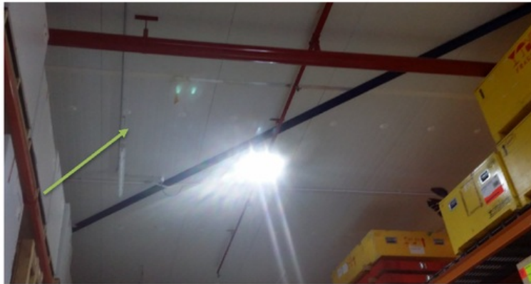
Figure 4.10. Detachment of vapour seal tape 5 in the ceiling panel joint.
