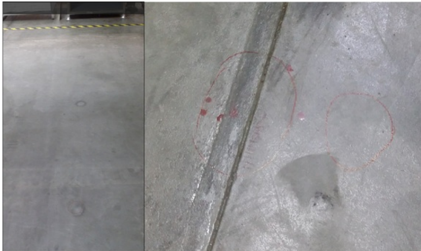
Figure 4.5. Condensation marks on the floor marked by personnel.
