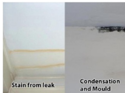
Figure 2.1. Example of deterioration of materials by leakage and condensation [14].
