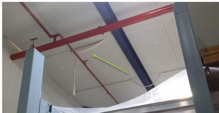
Figure 4.7. Detachment of vapour seal tape 2 in the ceiling panel joint.
