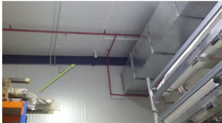
Figure 4.9. Detachment of vapour seal tape 4 in the ceiling panel joint.
