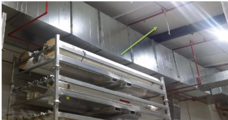
Figure 4.11. Detachment of vapour seal tape 6 in the ceiling panel joint.
