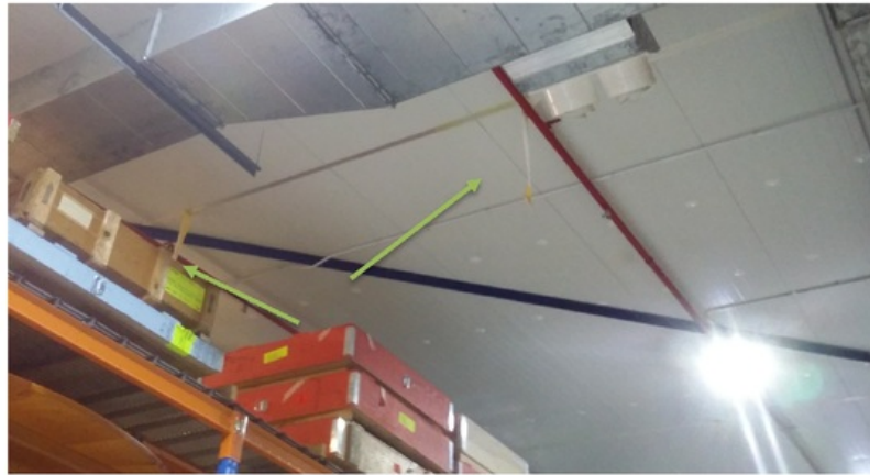
Figure 4.8. Detachment of vapour seal tape 3 in the ceiling panel joint.
