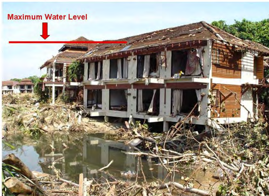
Figure 5.4: Maximum flow depths in Khao Lak reached 7 to 8 metres
