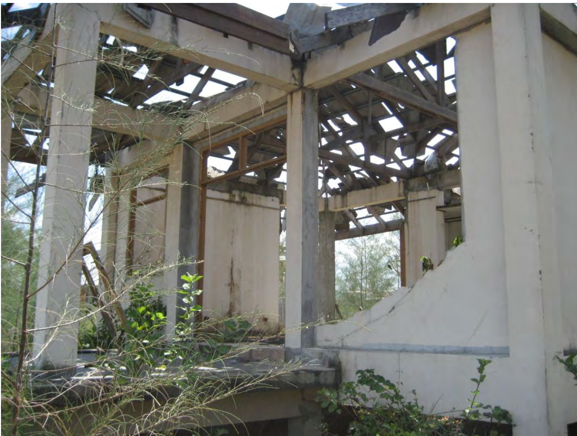
Figure 5.16: A house at Laem Pakarang exhibiting collapsed masonry infill walls with RC frames intact
