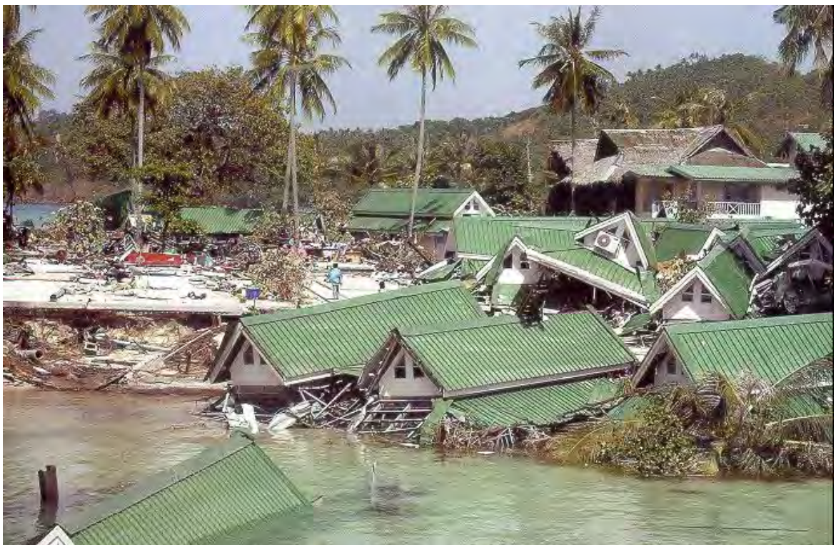
Figure 5.15: Collapse and displacement of wooden bungalows situated along Tonsai Bay, Phi Phi Don
