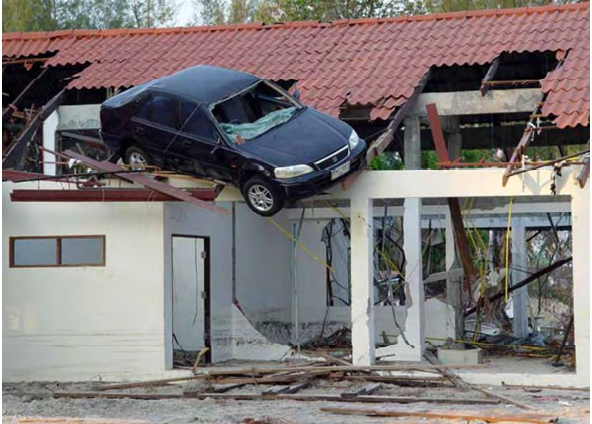
Figure 5.17: A car lodged in the roof of a damaged masonry building in Laem Pakarang, Khao Lak
