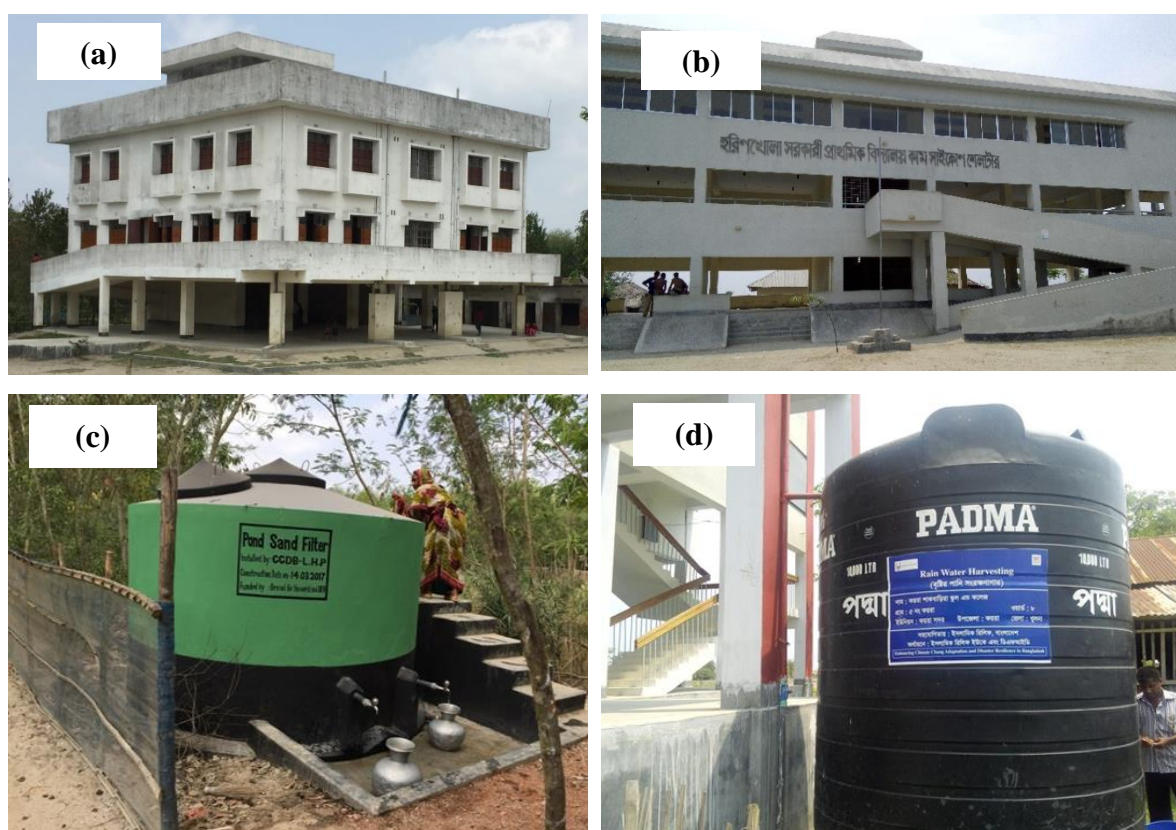
Fig. 6.8 Some representative pictures showing adaptation and mitigation measures: (a-b) school cum cyclone shelter; (c) Pond Sand Filter (PSF) for drinking water; and (d) Rain water harvesting tank.
