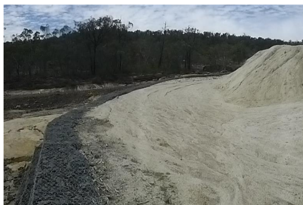
Fig 19: Transported tailings overtopping the containment of the LT before capping (29°57'2.82'' S 151°0'59.9'' E).
