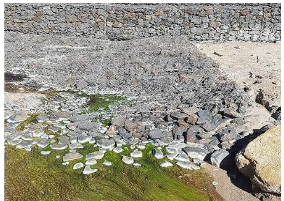
Fig 18: Efflorescence and algae amongst the discharge of the LT compound (29°57'1.99'' S 151°0'59.78'' E).
