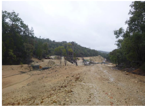
Fig 8: Haul road top dressed with waste rock (29°57'17.98'' S 151°1'33.16'' E).
