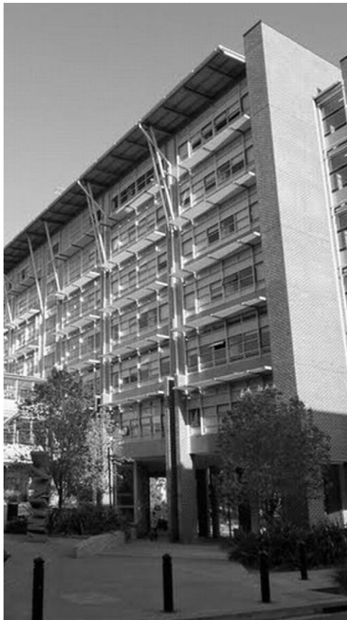
Fig. 1. MM building (Sunny/north facade) featuring operable windows with external solar shading devices on north-facing windows.
