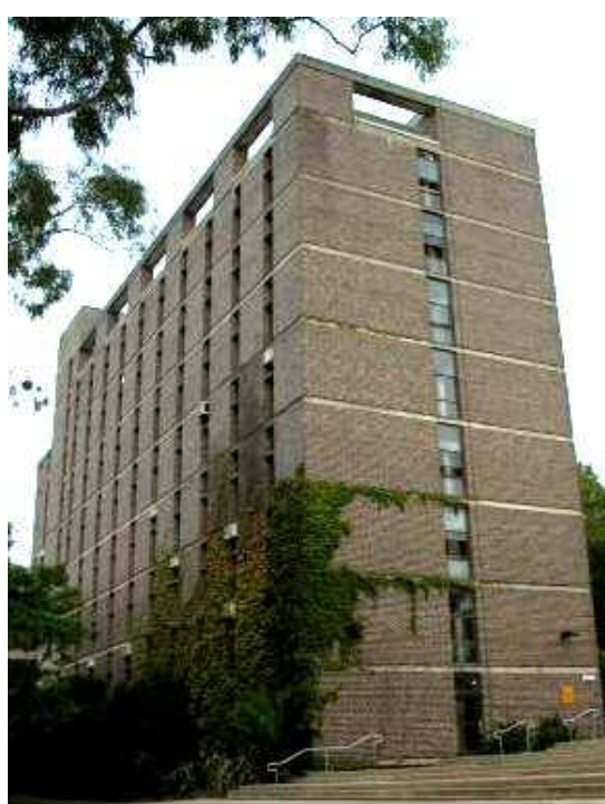
Photo 2: MQ, NV building (North façade) featuring occupant-operated windows with some individual air-conditioner units
