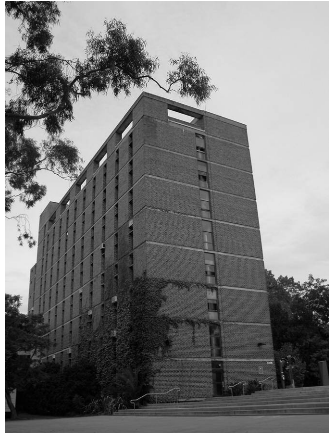
Fig. 2. NV building (North facade) featuring occupant-operated windows with some individual air-conditioner units.
