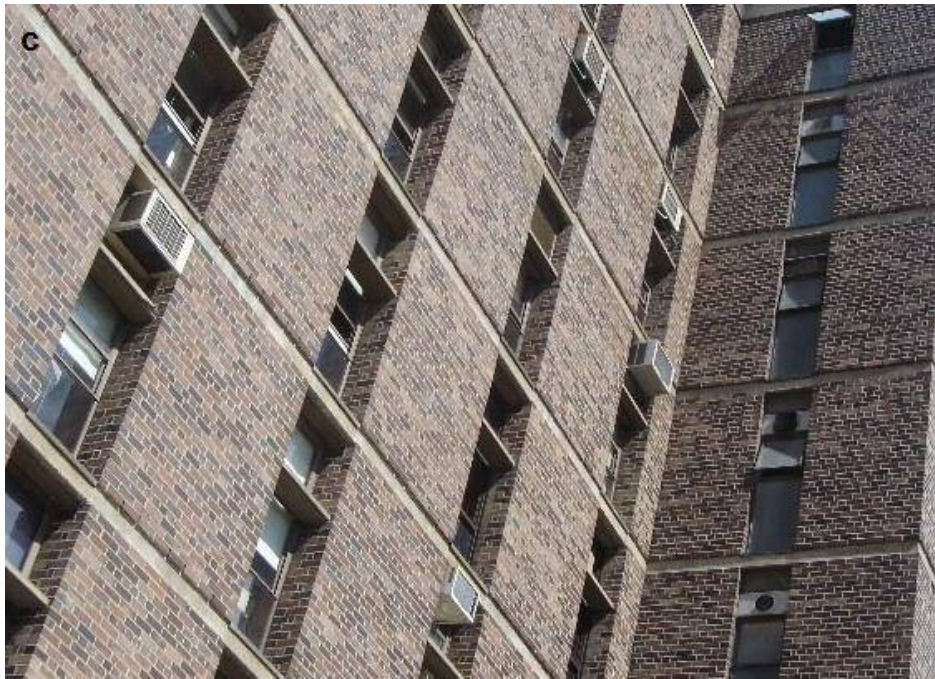
Figure 3.7c: Part of the North façade of Building E7A showing some offices with room air-conditioning units installed. The photo also shows ventilation fans in the windows of the toilets in the east-facing wall of the “dog-leg” of the north façade.
