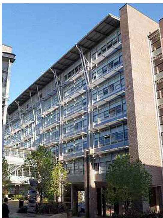
Photo 1: MQ, MM building (North façade) featuring operable windows with external solar shading devices on north-facing windows
