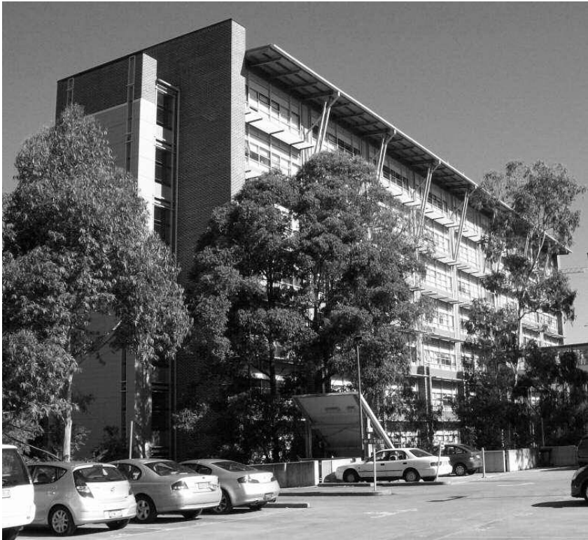
Figure 2a) The MM building as viewed from the north facade featuring operable windows with external solar shading devices on north-facing windows
