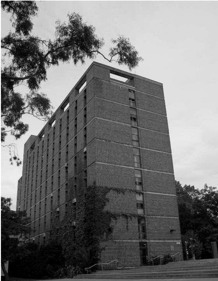
Figure 3a) The NV building as viewed from the north facade featuring occupant-operated windows with some individual air-conditioner units
