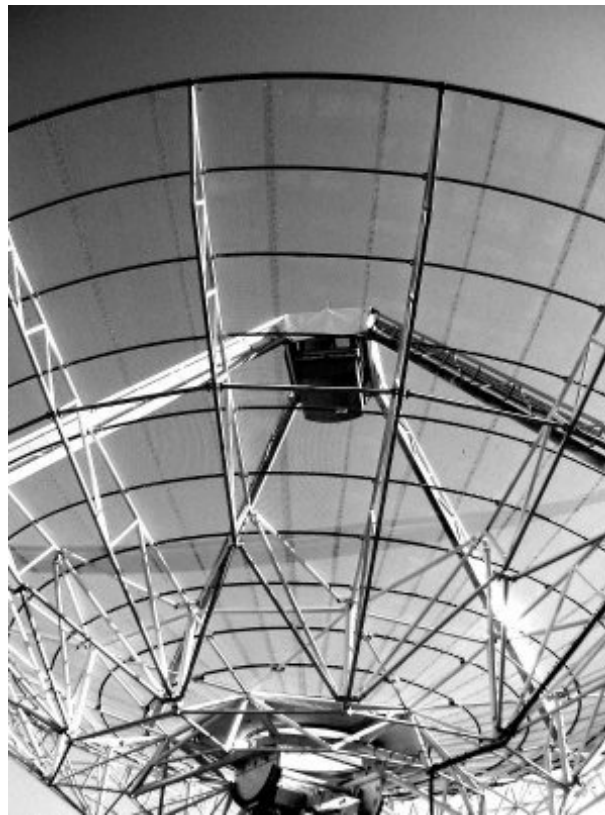
Figure 8.3 – NTD reflector: the reflector was constructed by fixing radial mesh panels to pipes formed into rings.
