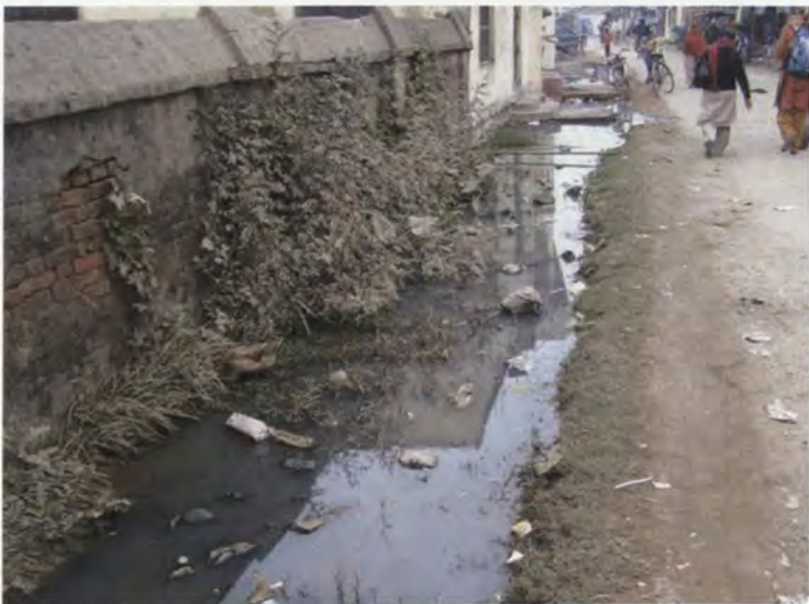
Photo 7.2 An example of a polluted and blocked drain in Nepalganj, Nepal. In recent years Nepalganj has experianced increased flooding from intense rain events and poor infrastructure to deal with runoff (Philip Ireland, 2010)
