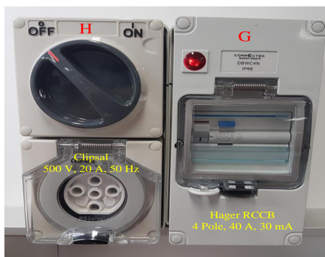
Figure 6.13. RCCB and main grid supply-pin outlet connections
