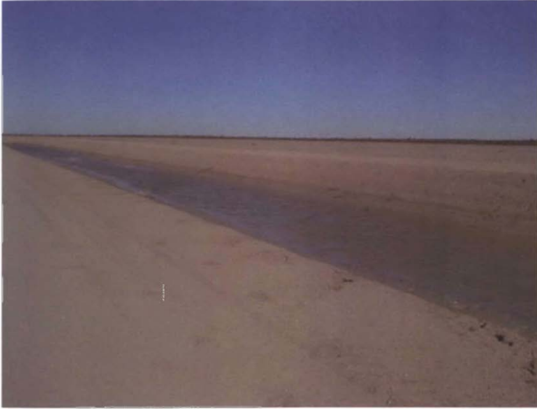
Plate 1 Temporary Irrigation Channel: Fed from the Namoi River
