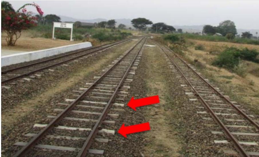
Plate 64: The track consisted of about one-third concrete sleepers and two-thirds wooden sleepers.
