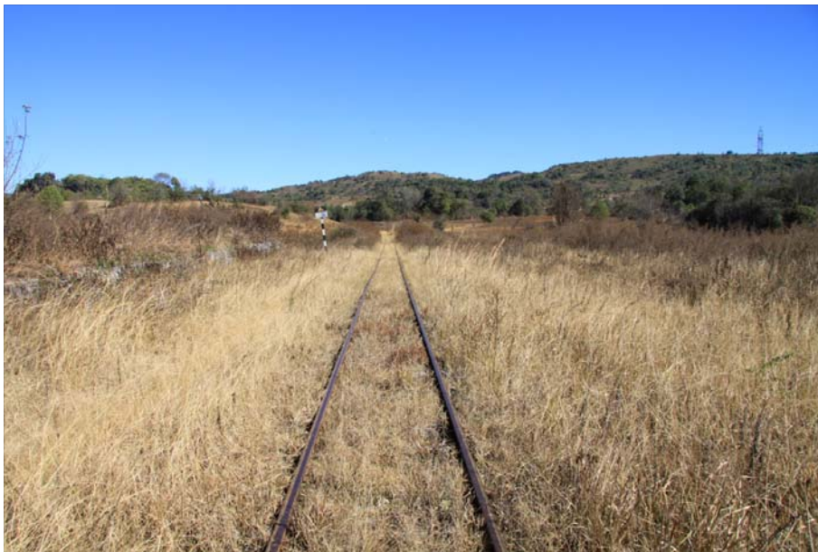
Plate 103: The track at Wa Lee is badly overgrown by weeds.
