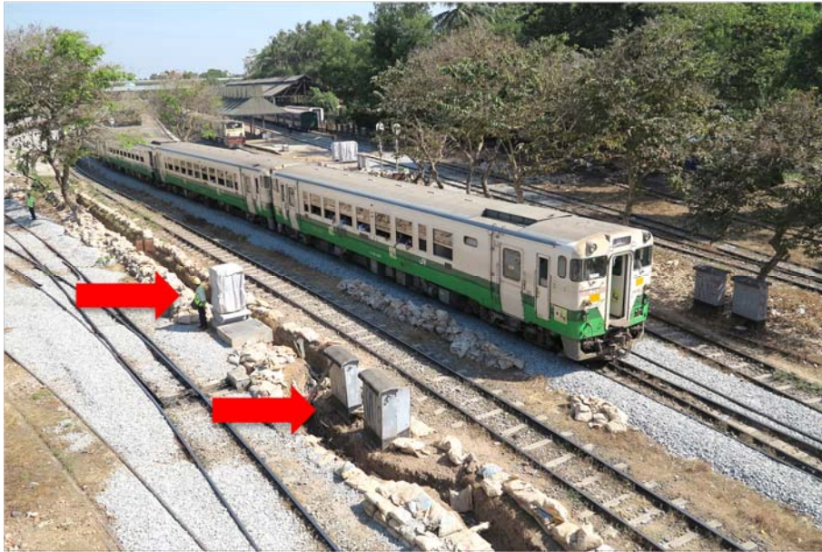
Plate 162: Signalling equipment being installed near Yangon Central Railway Station.
