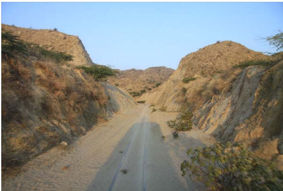
Plate 34: The line between Pakokku and Seikphyu, covered with dried mud and sand.
