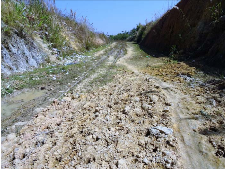
Plate 145: Track covered with mud in a cutting on the Shan State Railway.
