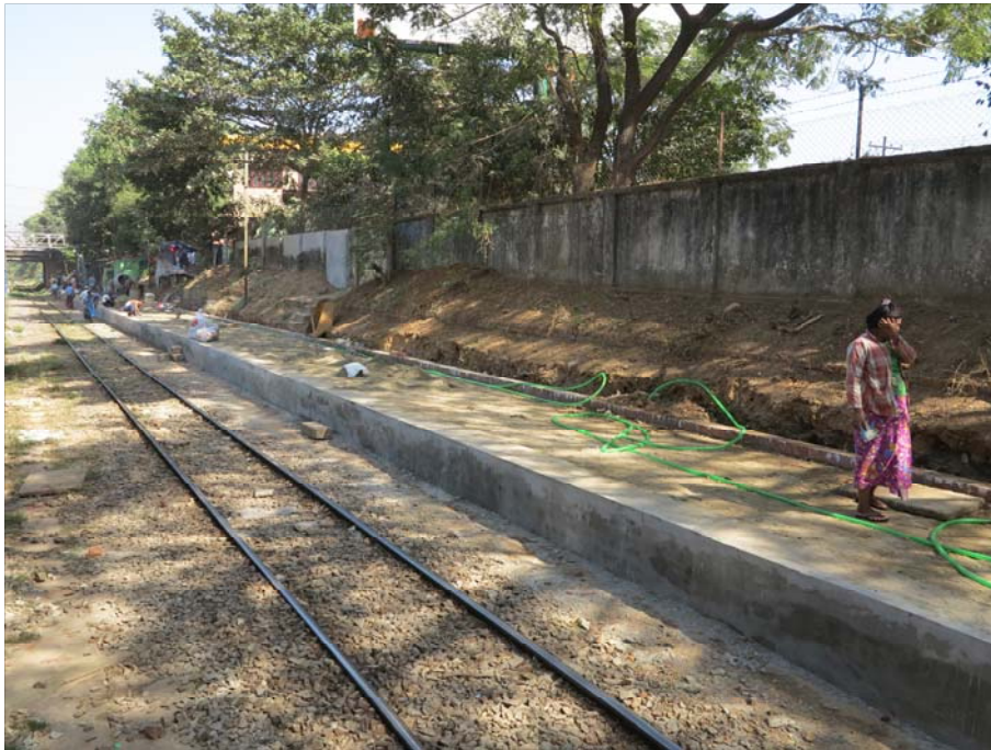
Plate 157: A platform being re-built at Kemmendine Station on the Circle Line in Yangon.
