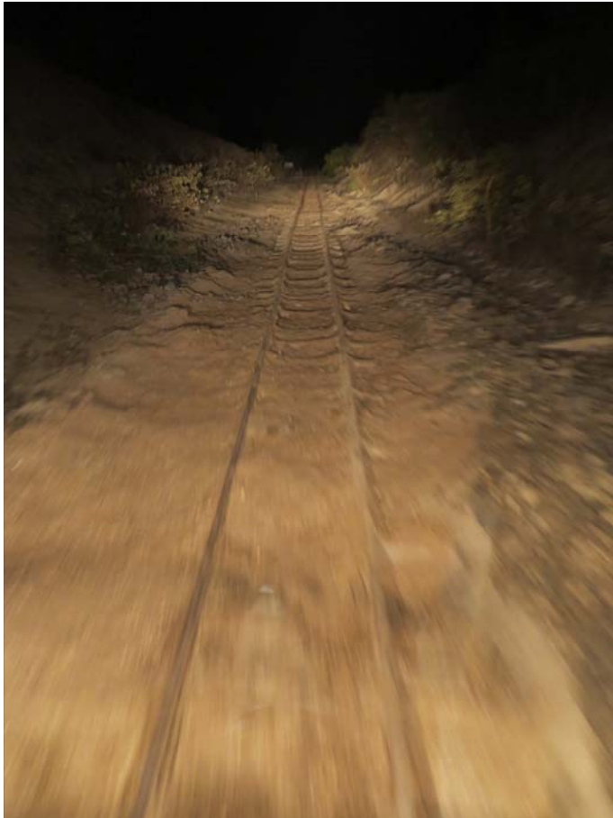
Plate 78: The track covered in mud and sand, with the rails barely visible.
