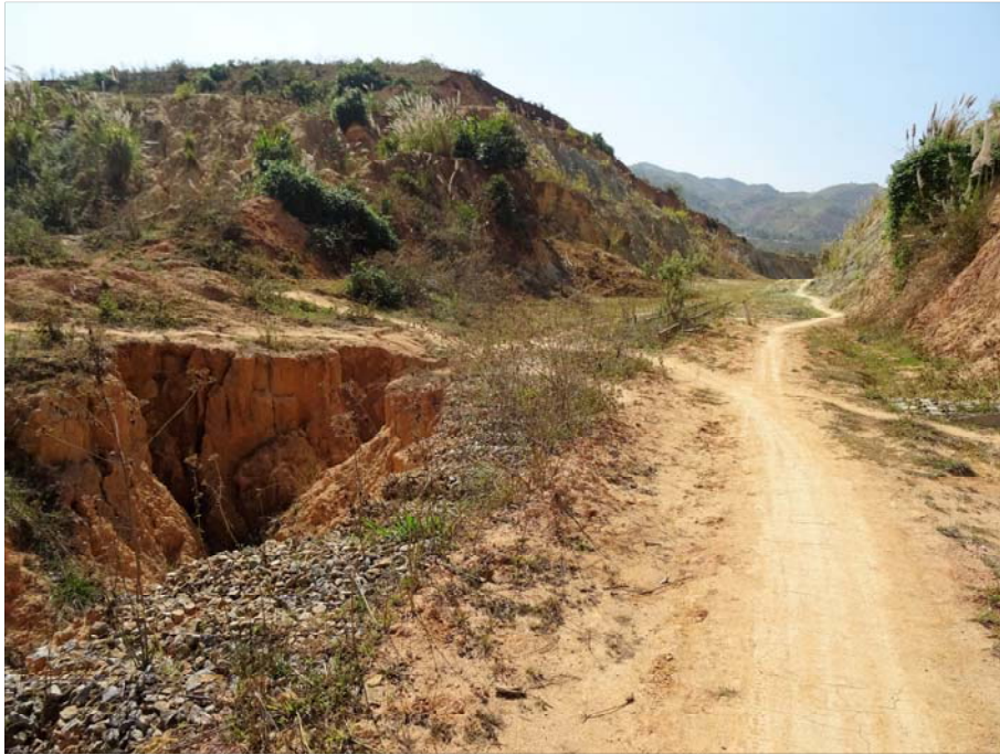
Plate 149: Badly eroded land along the track alignment.
