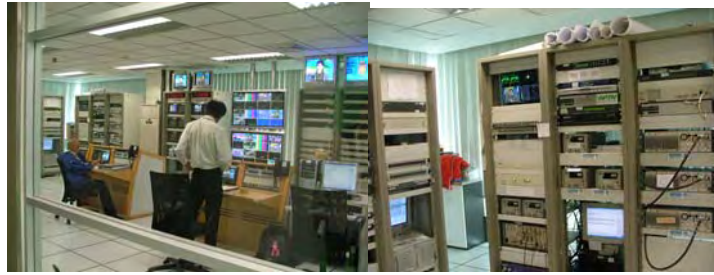
Picture 18 : A Broadcasting Operation Unit and Video Servers at Channel 3
