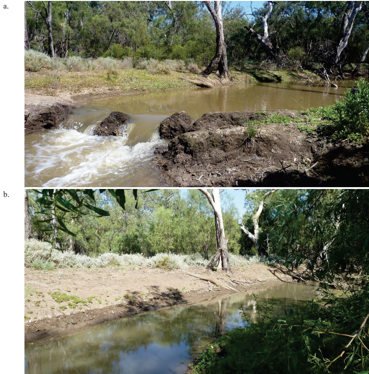
Figure 7.6 Macquarie River downstream of Bucklinguy Creek (SMM007) looking upstream in 2012 when the earth weir was present (a) and in 2018 (b) when the earth weir was absent. Photographs by Tim Ralph.
